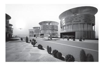
We are building low energy hangars to reduce electrical costs of heating or cooling in extreme climates, where the facade can house up to 850 photovoltaic panels.
